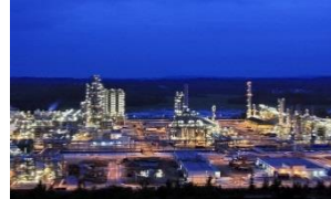
Dung Quat Refinery
