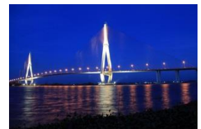
Can Tho Bridge
