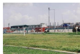
Nam Con Son Gas Treatment Factory
