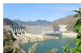
Sơn La Hydropower plant
