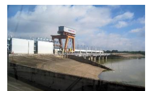
Trị An Hydropower Plant
