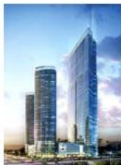
Keangnam Landmark 336m/1.132 ft Hà Nội, 2011 Main Contractor : Keangnam Enterprise Project Manager : Parsons Brinckerhoff
